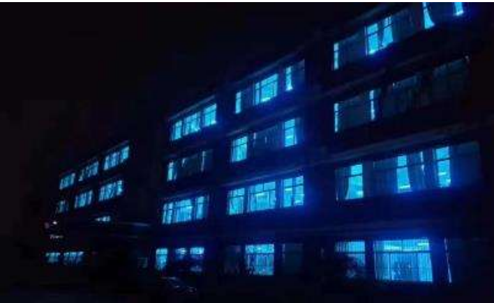
Office building in Wuhan Pulmonary Hospital
